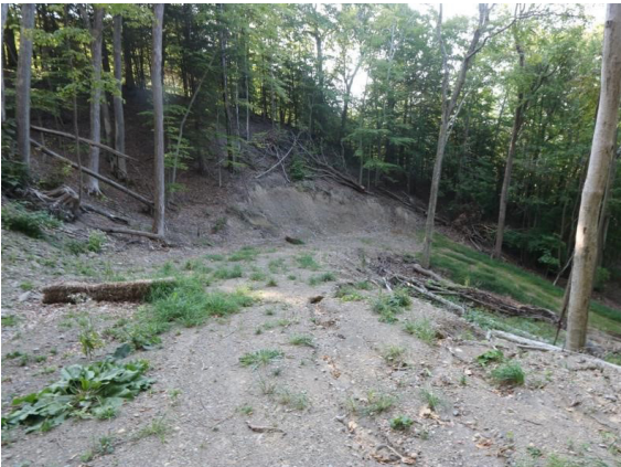
Esker repair - Photo credit: CNY Land Trust
